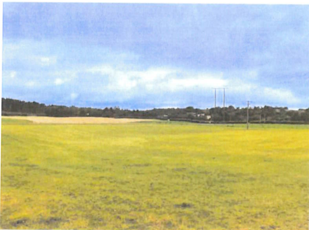
Figure 5. View across the central portion of the holding showing the existing 110kv overhead electricity transmission line.
